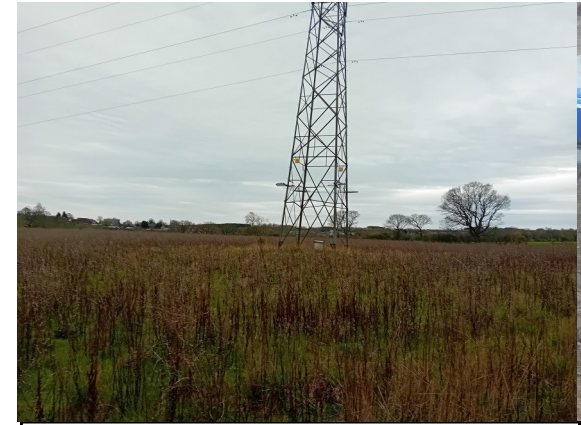
Photo 3— Pylon in NE field.
